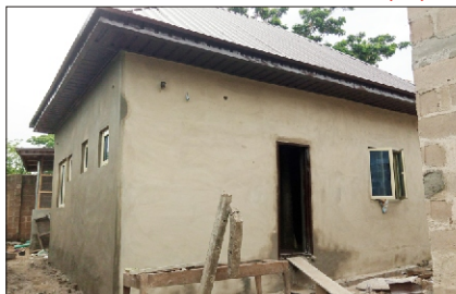
Renovation and expansion of Patient's Cafeteria at Lantoro Annexe
