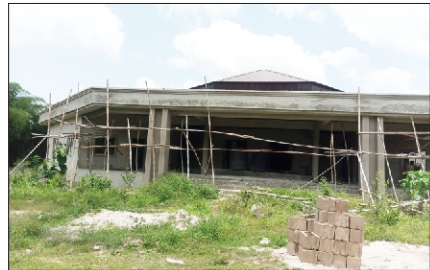
Construction of 250-Seater Auditorium at Aro
