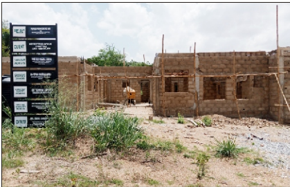
Construction of Psycho-geriatric Clinic at Aro
