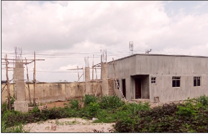
Construction of Second Gate at Aro
