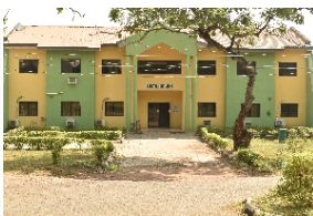
Research and Training Building
