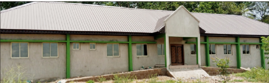
Construction of Multipurpose Physiotherapy Building at Aro
