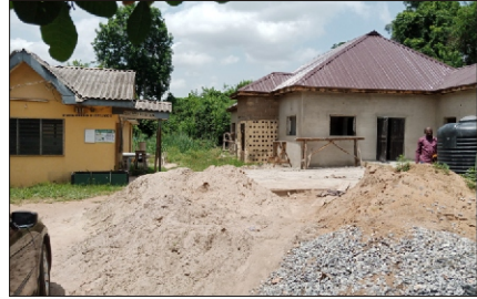
Renovation and Expansion of Mortuary at Aro
