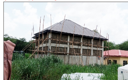
Construction of Oxygen Plant at Aro
